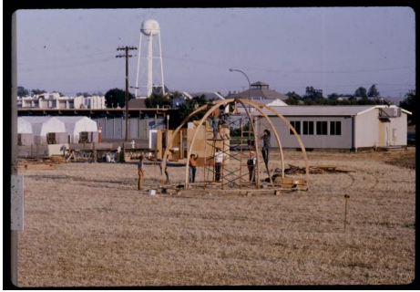
Making the frame for Dome mold
