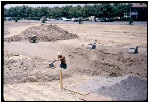
Digging the hole to hold the mold
