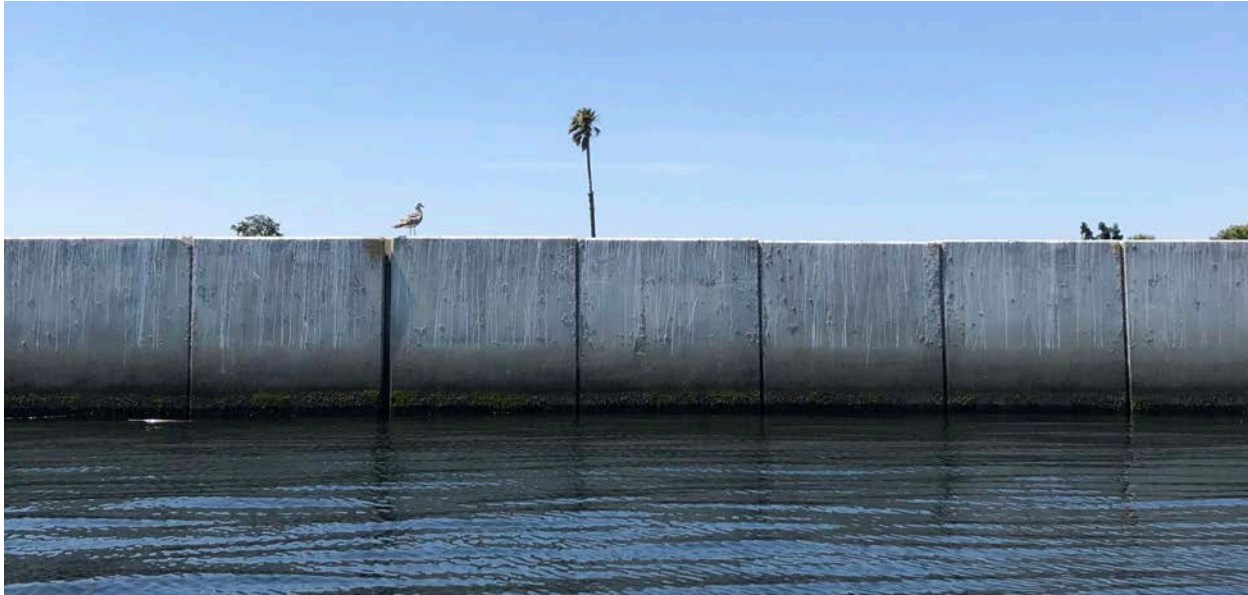
Concrete levee barrier, Franks Tract, 2018
