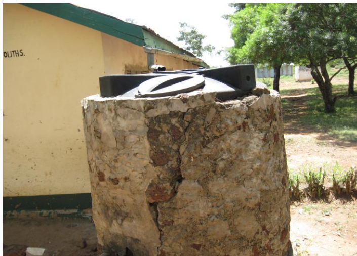
Plastic Rainwater Catchment Tank (Cement around the outside protects it from the sun.)
