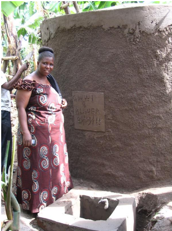
Ferro Cement Rainwater Harvesting Tank
